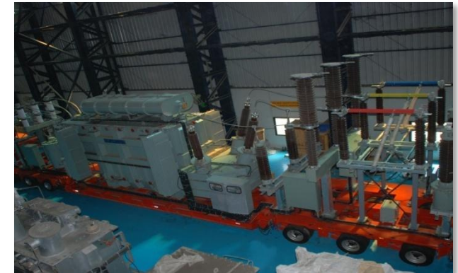
Substation - erection & commissioning
