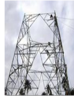
Transmission tower erection
